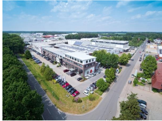
Image 2: More than 750 employees work for Vogelsang at the company headquarters in Essen (Oldenburg).
